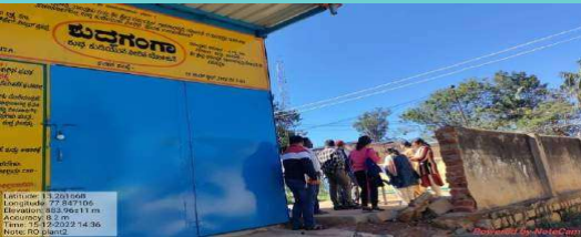
RO Plant, Jangamakote village
